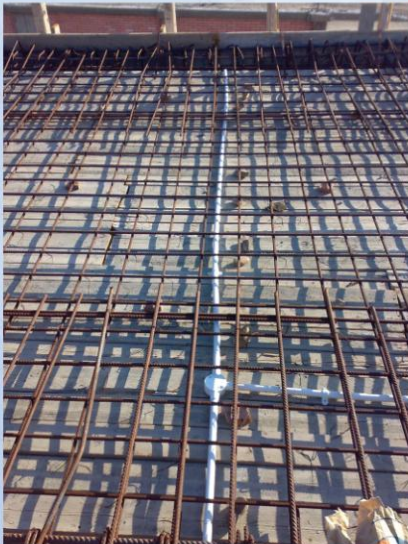
Installation for Electrical systems inside adminastration building and control buildings
